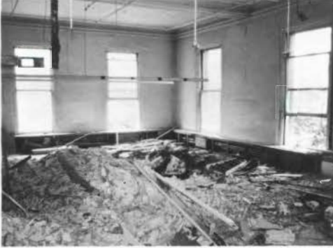
Through the generosity of alumni and friends, Lewisohn Hall was renovated in 1980–1981. This photo was taken neither before nor after, but during.
